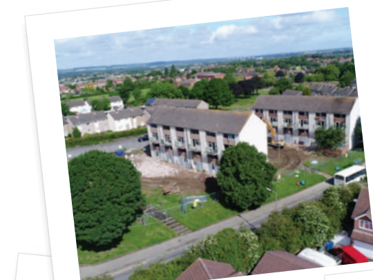
Tinkers Green demolition commences
